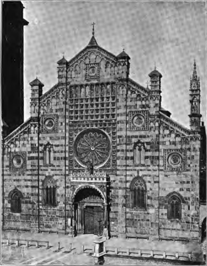
FAÇADE OF MONZA CATHEDRAL. RESTORED 14TH CENTURY. [To face page 380.
